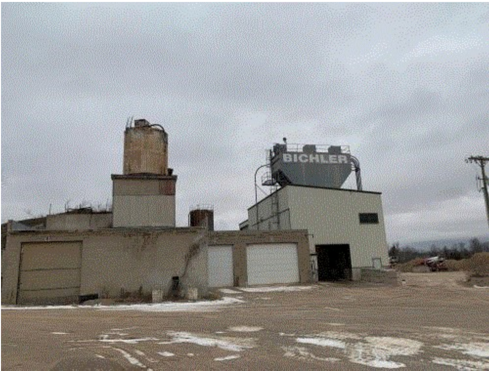
Image 3(Concrete Batch Plant) : Warehouse used for facility's concrete operations.
