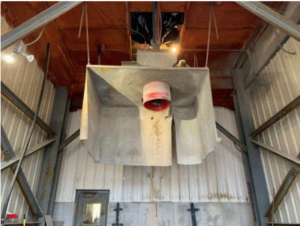
Image 4(Loading Chute) : Chute used for concrete loading.
