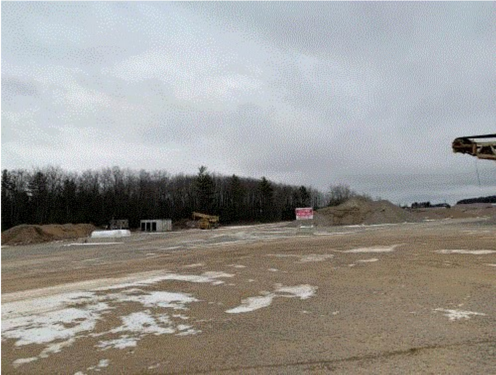
Image 2(Facility Yard) : Yard for truck traffic.
