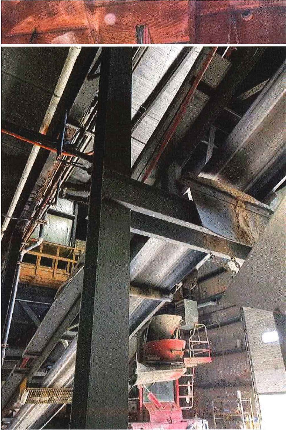
Image 3(Conveyor) : Conveyor to concrete dispenser
