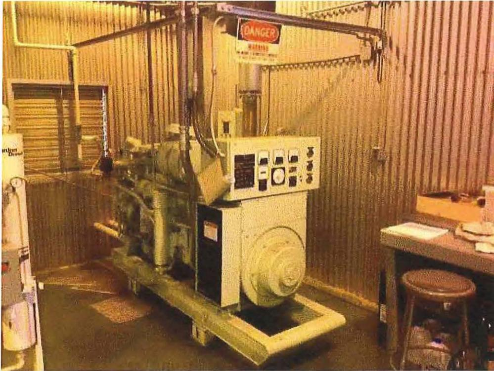
**Image 2(GLGT10A2) :** Emergency generator APU operates on natural gas
