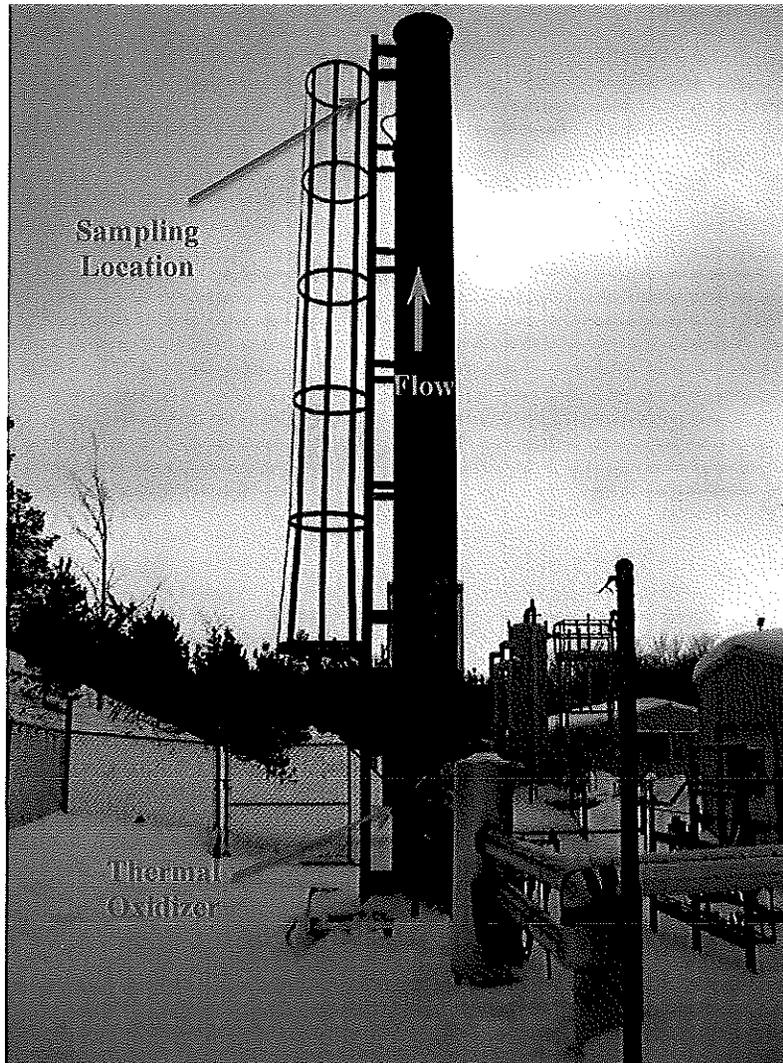
**Figure 2-3. Excelsior Thermal Oxidizer Exhaust Stack**
