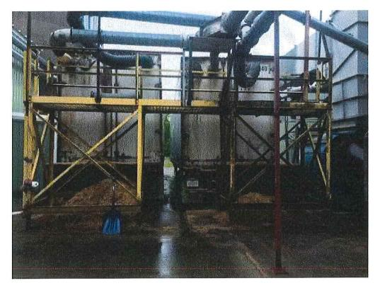
Image 2(Truck Trailers): Wood residue that is collected from the baghouse is routed to either the truck trailers or the silo in an enclosed system.
