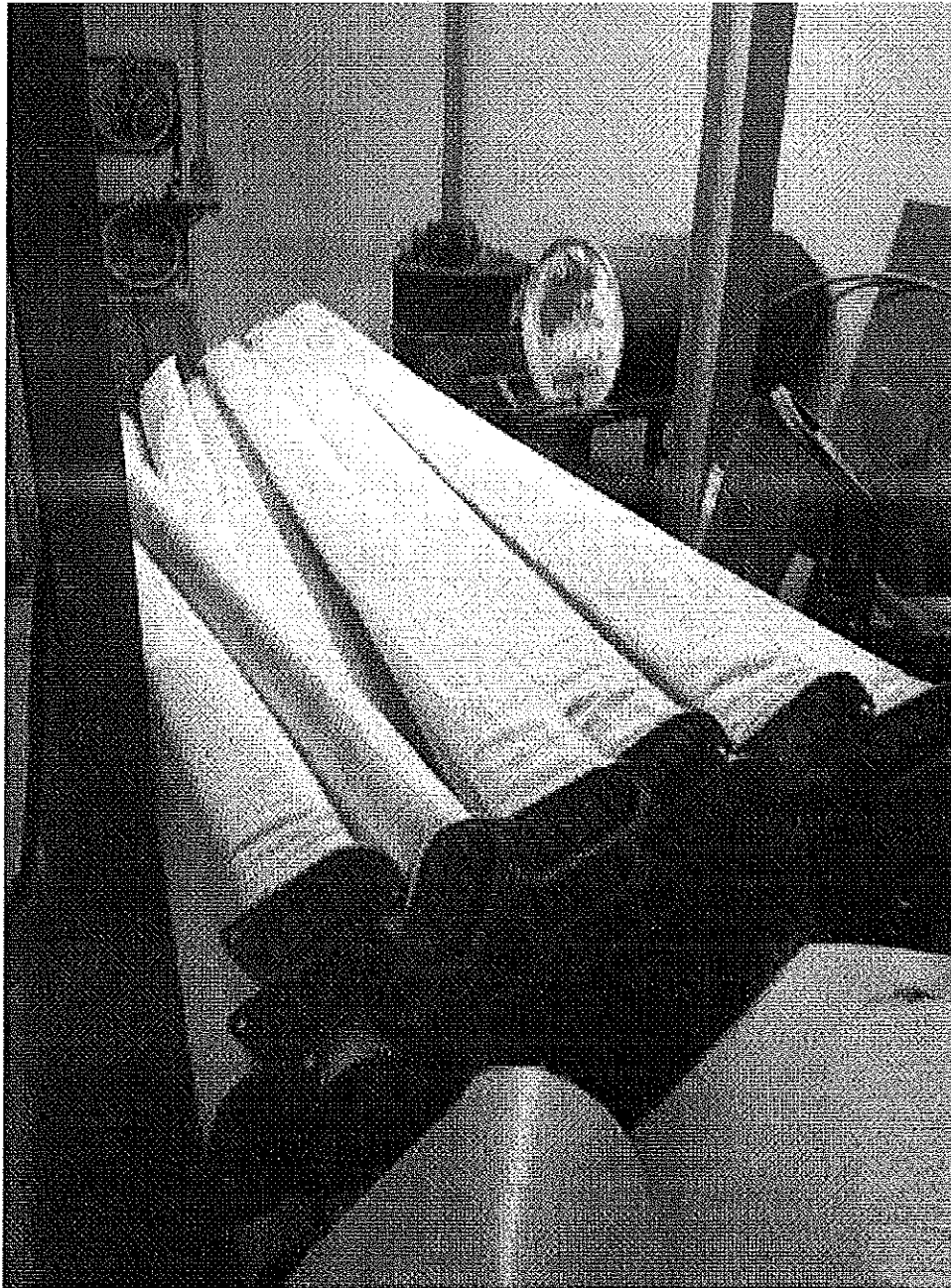
Image 9(7/24/2014) : Remaining new bags ready to be installed.
