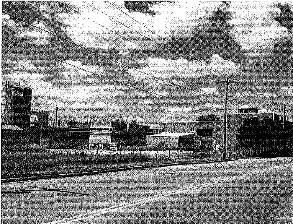
Image 1(7/24/2014) : Exterior view of facility. Waste storage silo, cyclone and boiler outbuilding can be seen on the left side of frame.
