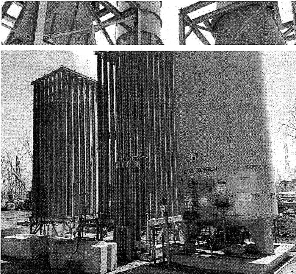
**Image 25(Oxygen tank-torch) :** Oxygen storage tanks for torch cutting
