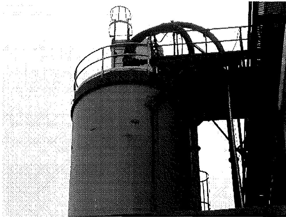
**Image 2(DSC00070)** : Photo of baghouse dust silo with bin vent to control fugitive emissions during truck loading.
