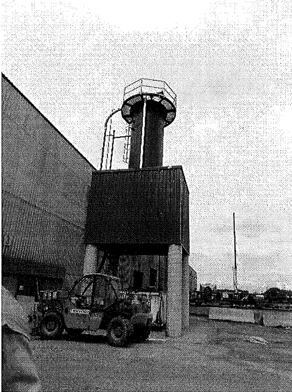
Image 8(DSC00091) : Photo of dust collection system for vacuum system serving the twin VTD's
