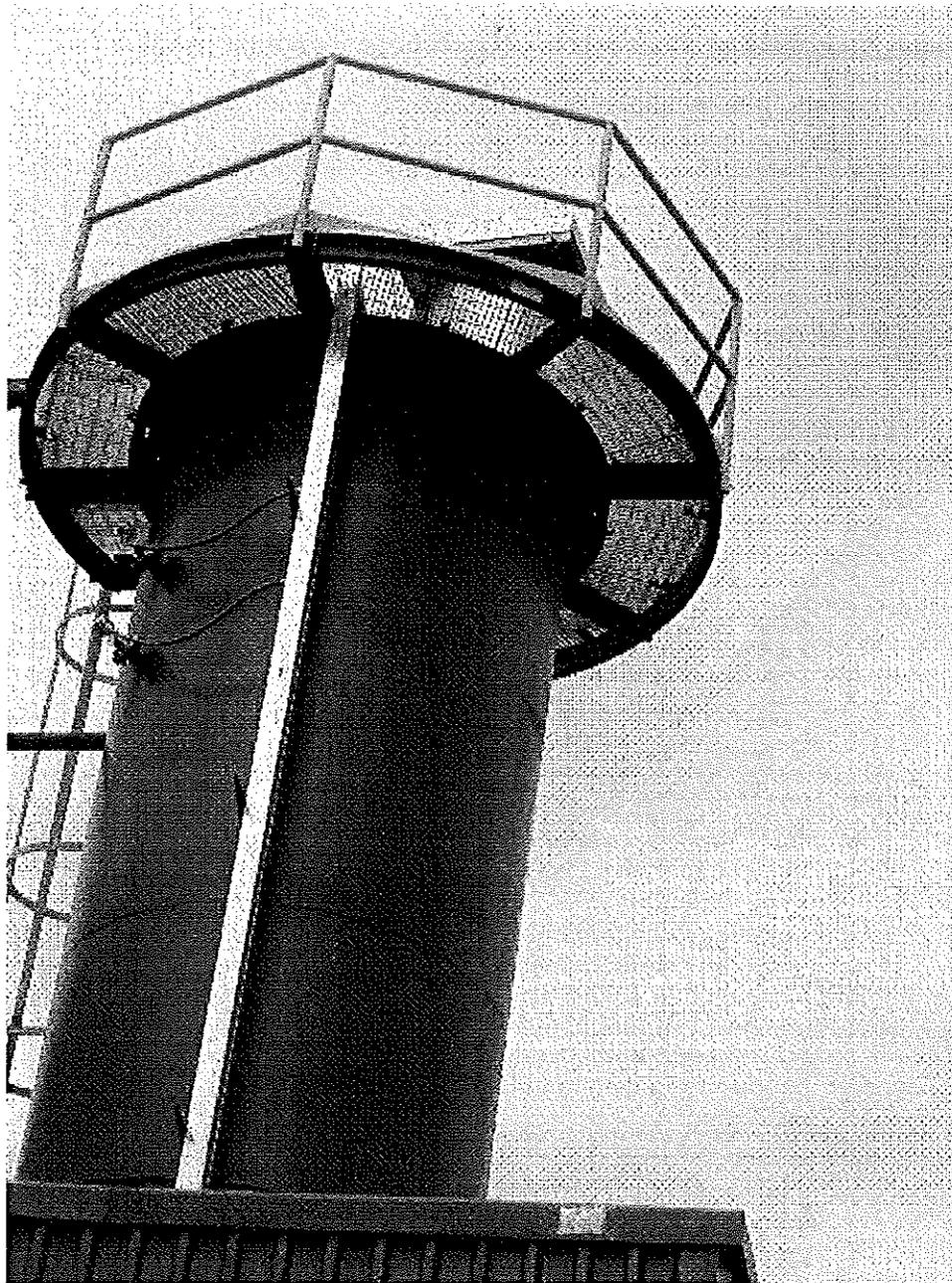
**Image 9(DSC00092)** : Another view of the dust collection system for the vacuum pumps serving the VTD's
