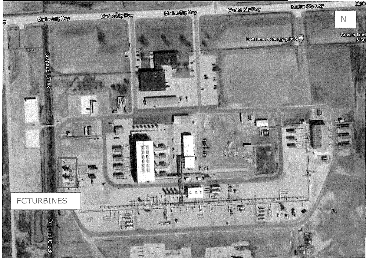
Figure 3-2. St. Clair Compressor Station Plant 1 Turbine Location
