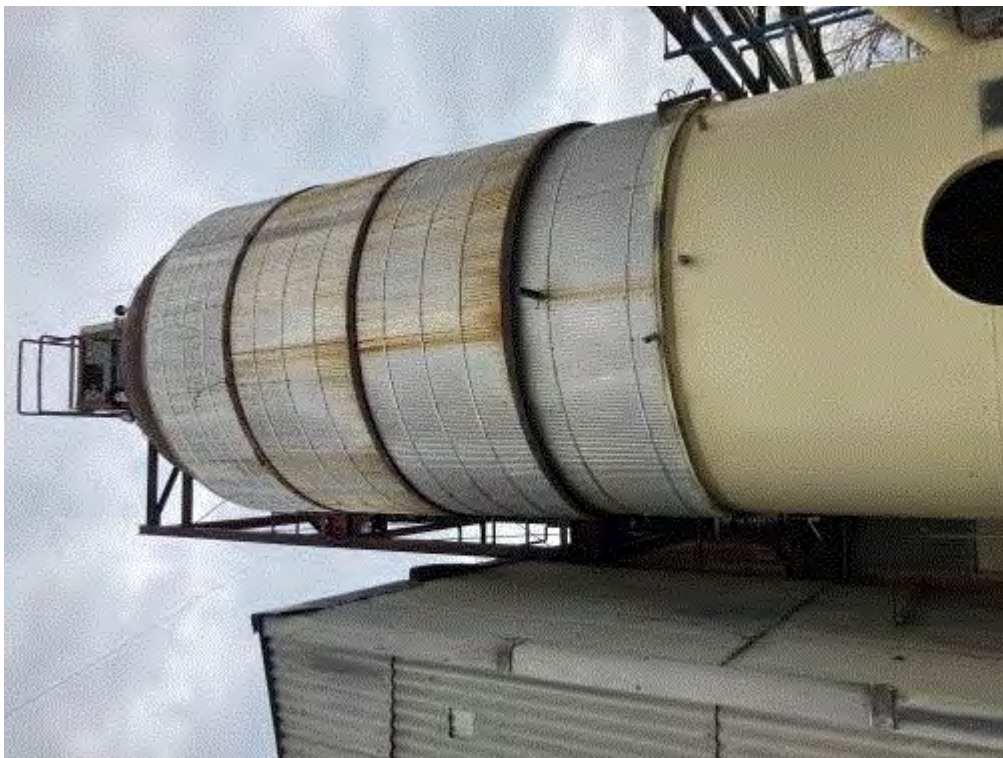
Image 3(003) : Lime storage silo EULimeTank540 on 4/13/2022.
