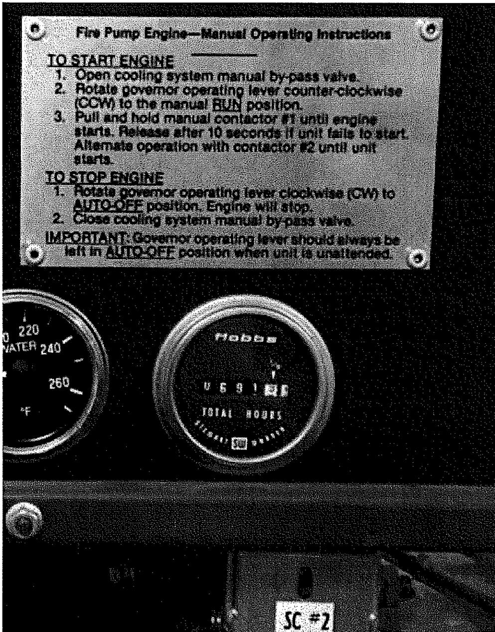
**Image 9(9) :** West Clarke Detroit Diesel Pump 2 - Hour Meter from May 18, 2018. Photo supplied by Duke Couch
