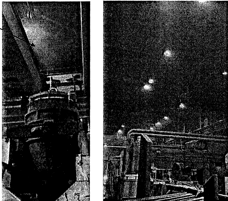
Figure 3.6 Emissions Generated at Caster (Left) / View from Caster Deck (Right)
