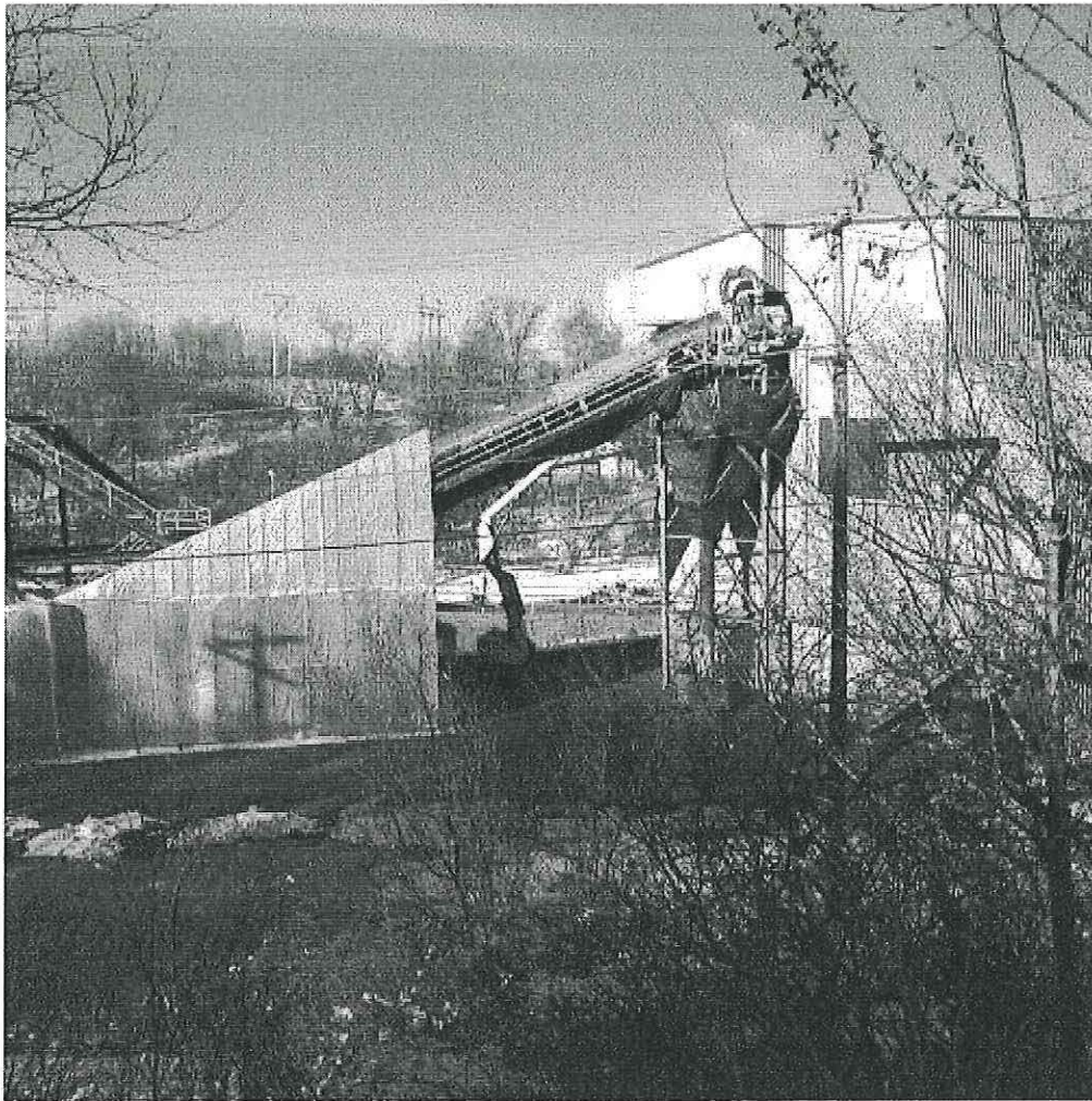
Image 1(Photo 1) : LWEC incline conveyor. Photo taken on March 21, 2016.
