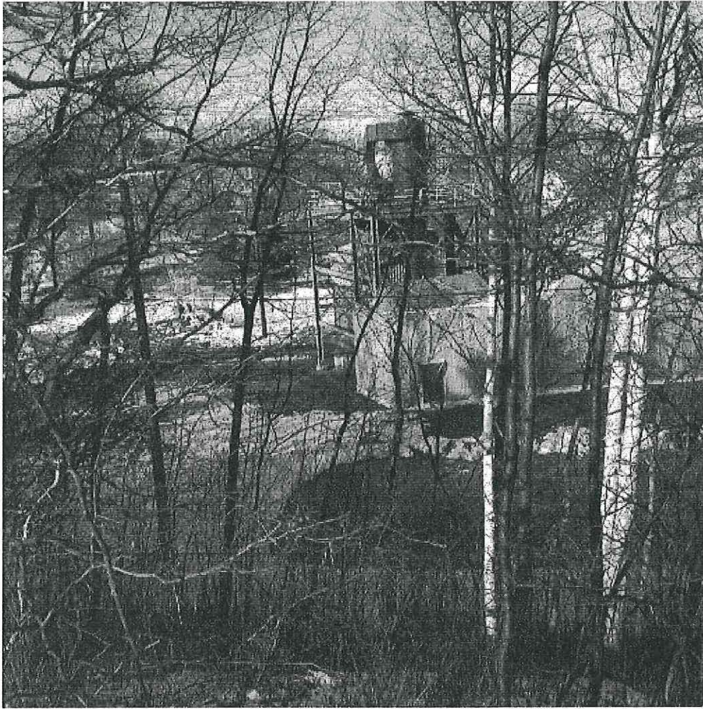
Image 2(Photo 2) : LWEC fuel receiving hopper. Note build-up of dust on hopper structure. Photo taken on March 21, 2016.
