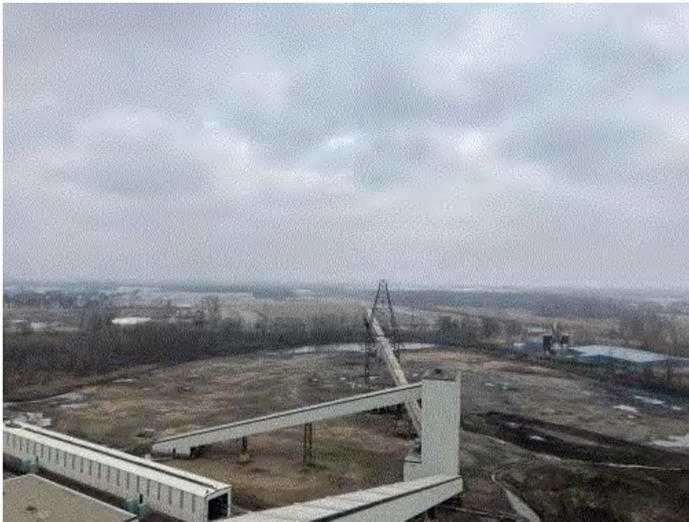
Image 1(11) : Coal conveyors to be removed and ash handling building in background.
