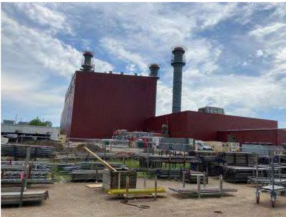
Image 6(0191) : DEP under construction
