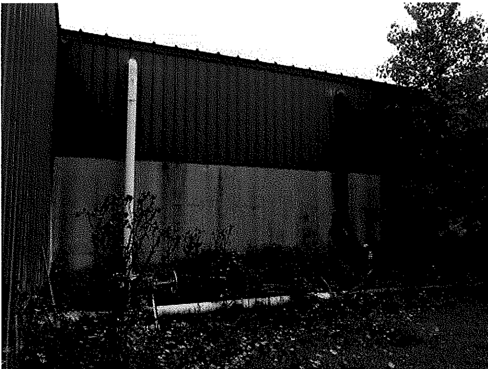
Image 4(Pneumatic Piping) : A portion of the pneumatic fly ash piping system entering the mass storage building
