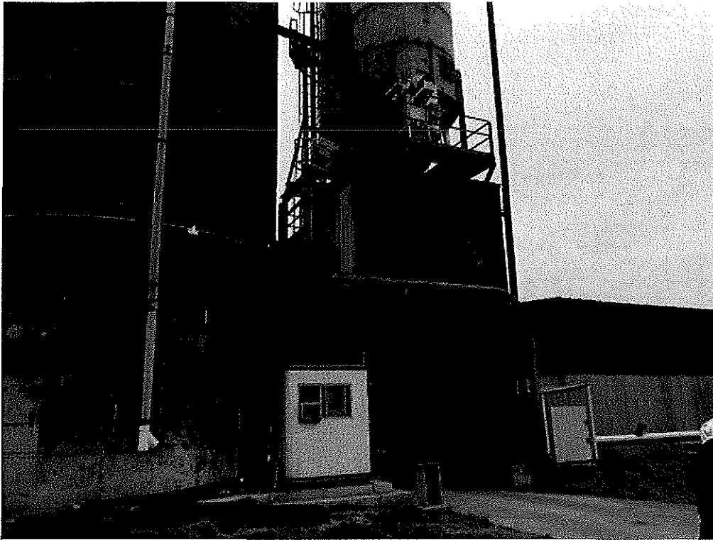
Image 7(EUASHDC3) : Truck loadout silo chute baghouse (small white unit located near the base of the silo)
