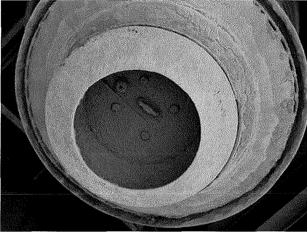
Image 2(FGASHHANDLING) : Fly ash loadout chute with new seals
