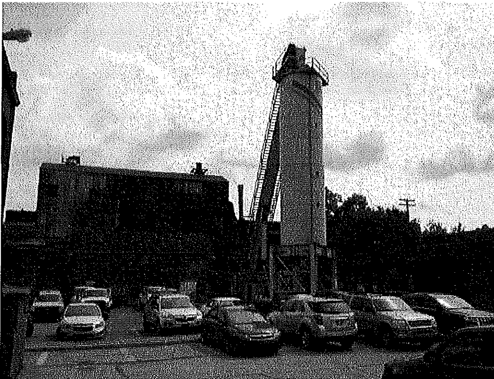
Image 1(asphalt production) : Idled, permanently shut down asphalt production facility.
