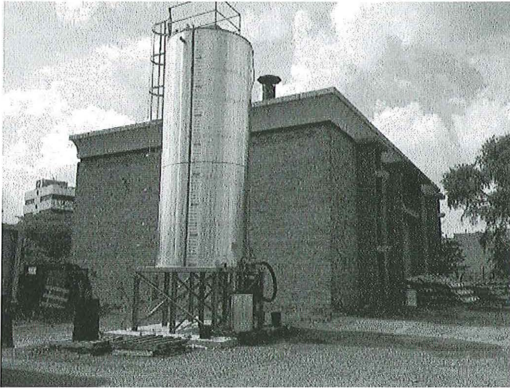
Image 2(emulsion tank) : New 8,000 gallon capacity asphalt emulsion tank (electrically heated).
