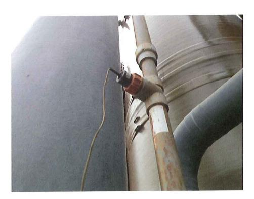
Attachment 3—Photographs of (1) Flow Meter FM502-1 and (2) Display— Installed on Second Stage (Tower II) of Two-Stage Scrubber
