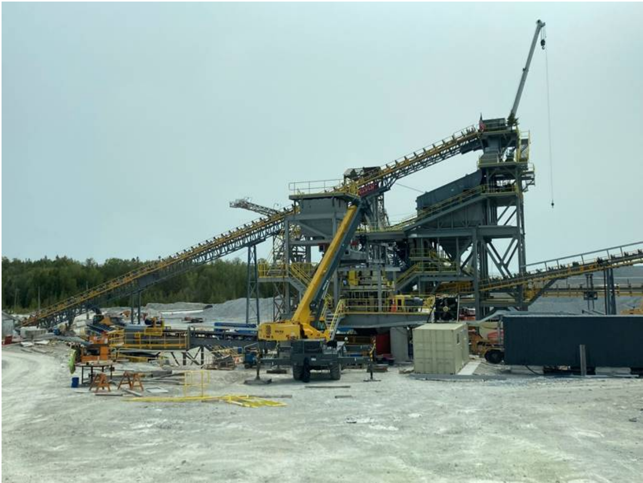
Image 1: Equipment under construction
