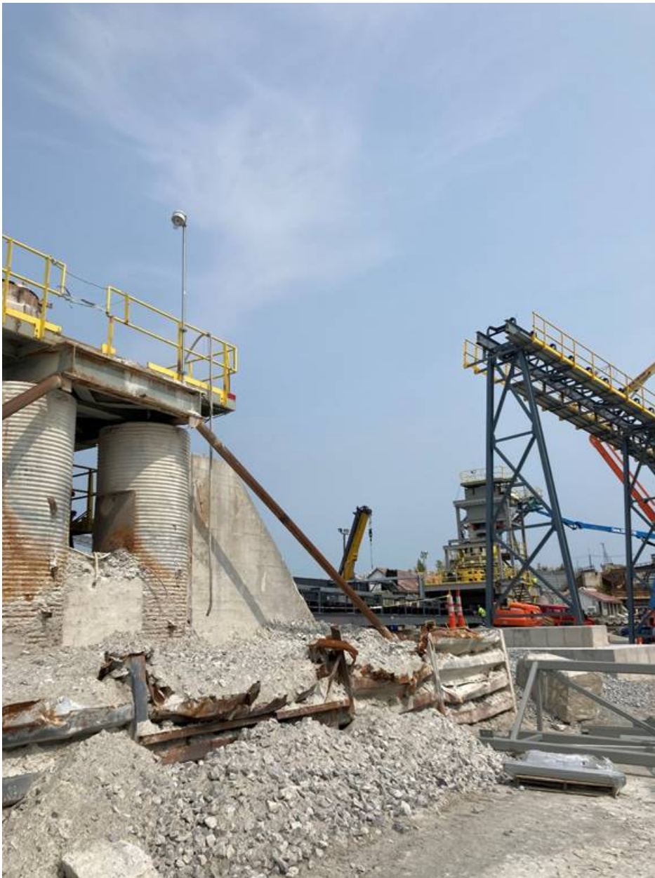
Image 2: Equipment under construction
