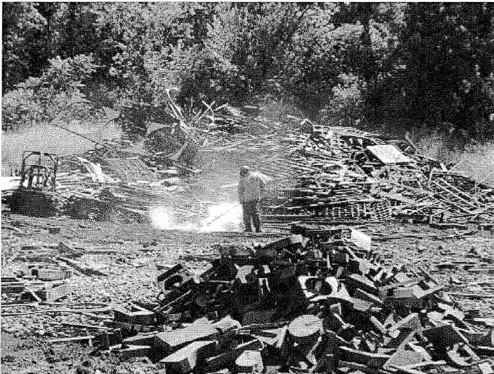
**Image 12(Figure 12)** : Torch-cutting operation (8/3/2015, 11:26 am).
