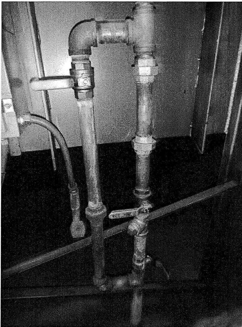
**Image 5(Figure 5) :** Venturi Scrubber water supply valves, in the "off" position. The facility confirmed that the water supply was turned off, as they add water manually, as needed (8/3/2015, 10:37 am).
