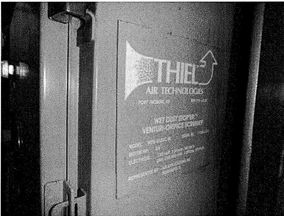
**Image 4(Figure 4) :** Venturi scrubber make and model plate. Thiel Air Technologies, Wet Dust Stop'er Venturi-Orifice Scrubber, Model WDS-0S22C-BL, Serial Number 1104-2366 (8/3/2015, 10:36 am).
