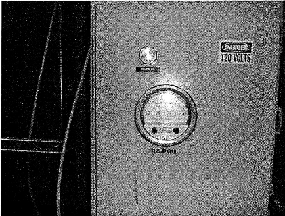
**Image 3(Figure 3) :** Venturi scrubber sump level gauge (8/3/2015, 10:36 am).
