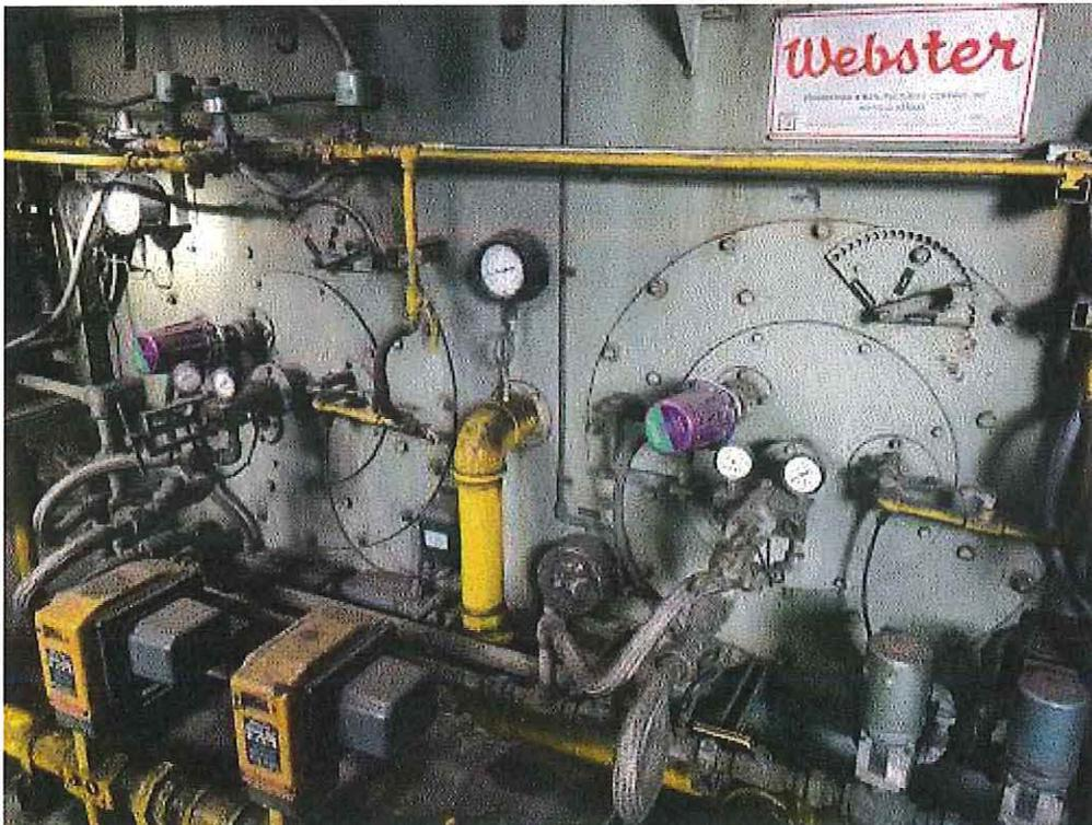
**Image 6(EUBOILER1)** : Natural gas-fired boiler with a rated steam capacity of 70,000 lbs/hr.
