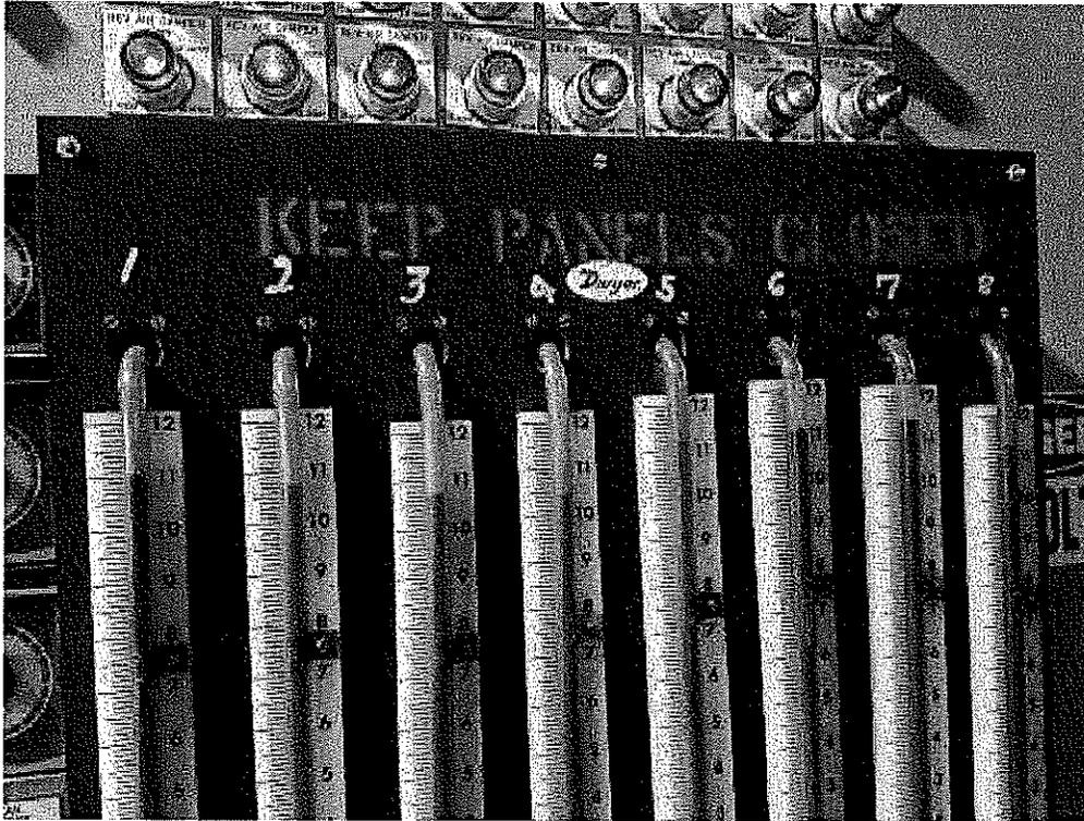
**Image 4(EAF Baghouse Press.) :** EAF Baghouse pressure differential for each of the 8 compartments. Shows 10 to 11".
