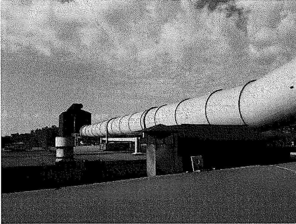
**Image 6(EAF Baghouse Vent.)** : EAF baghouse ventilation pipe from roof.
