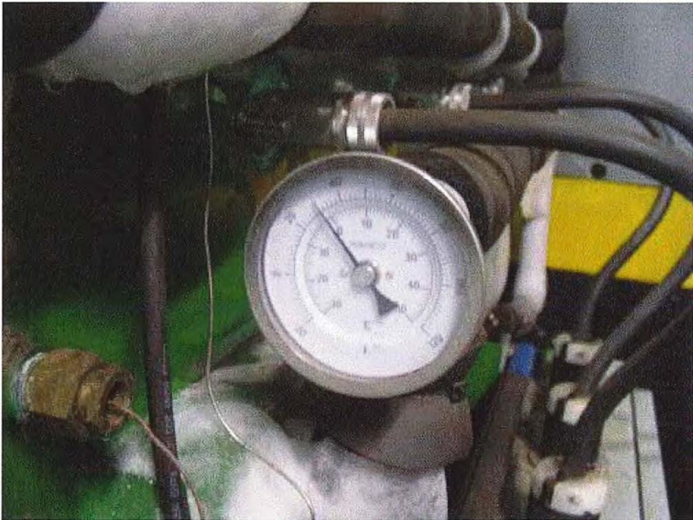
**Image 6(006) :** Chiller outlet for lower level coils.
