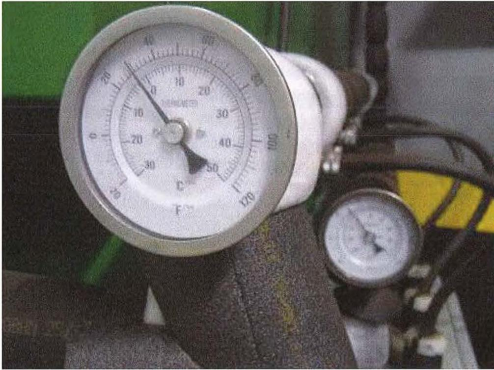
Image 4(004) : Chiller inlet temperature gauge.
