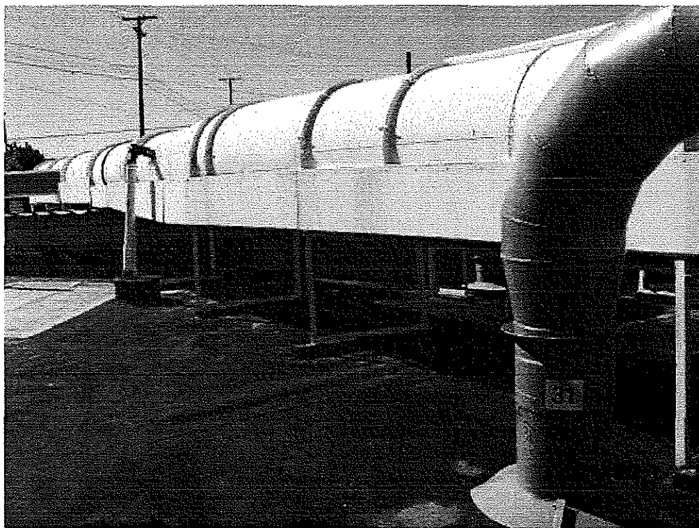
Image 3(Photo 3) : Scrubber #3 ductwork, looking SE.
