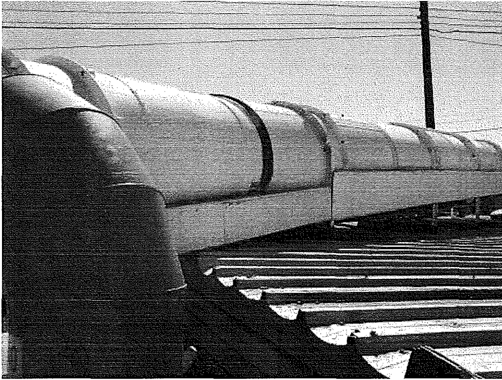
Image 5(Photo 5) : Scrubber #3 ductwork seen from west side, at south roof.
