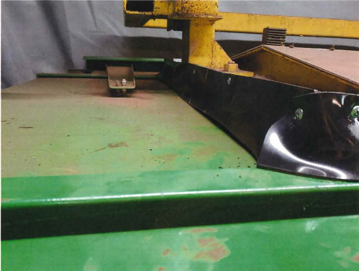
Photo 7: View of rubber shield installed on November 1, 2019 to cover gap between working mode cover and degreaser.
