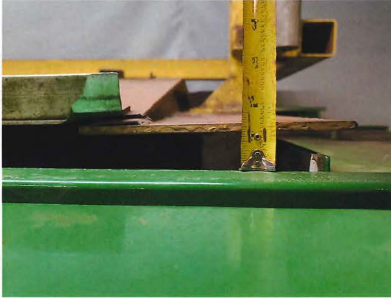
Photo 3: View of approximate 1-inch gap between the working mode cover and degreaser.
