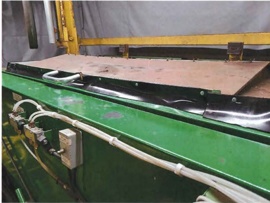
Photo 5: View of rubber shield installed on November 1, 2019 to cover gap between working mode cover and degreaser.
