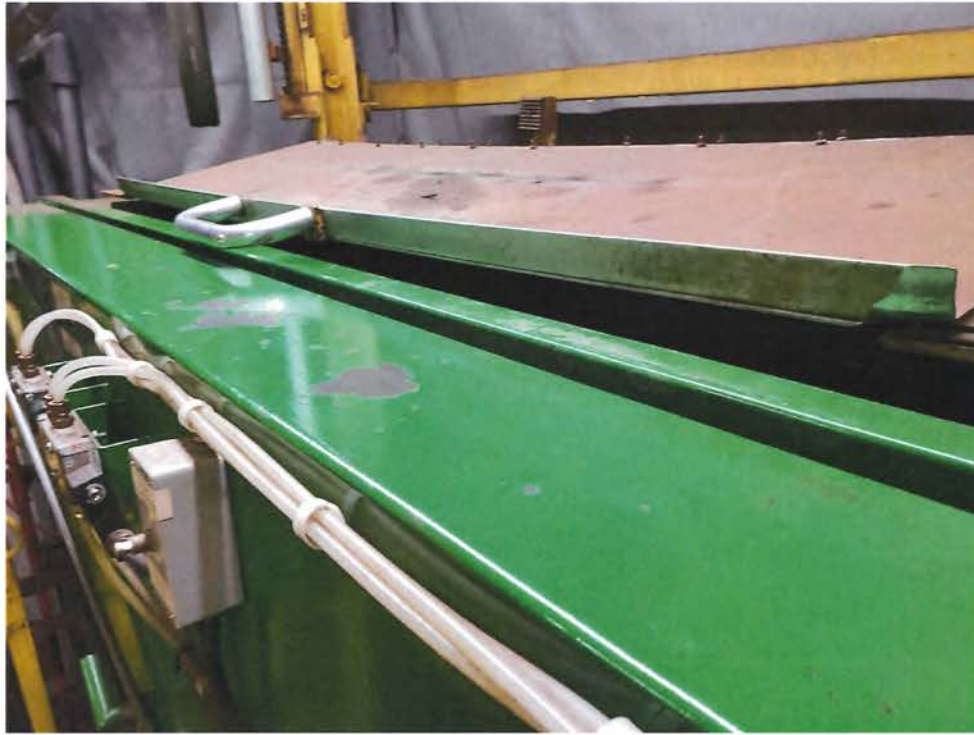
Photo 1: View of approximate 1-inch gap between the working mode cover and degreaser.
