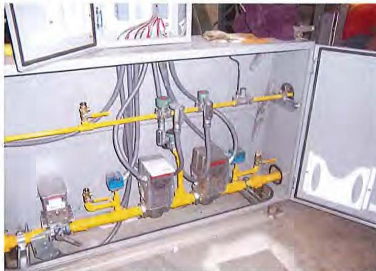
Photo shows a piped gas train mounted inside a weather-proof enclosure
