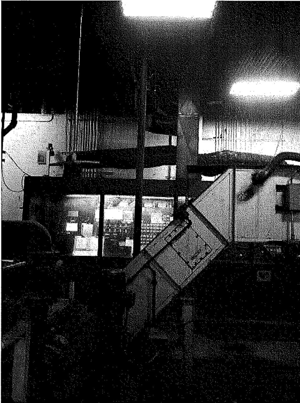
**Image 2(Figure 2) :** Observed smoky emissions emanating from EU1CHARDENTEMPE's temper furnace during the inspection. Some emissions were not captured by the hood and routed outside via the stacks.
