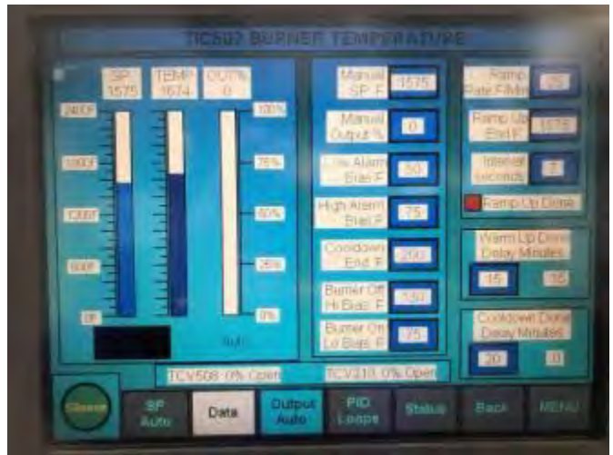
Burner temperature overview screen online. Customer would like to have PID setting check might need change program
