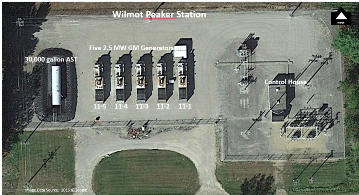
Figure 1-1. The facility consists of five 2.5 MW generators, a 30,000 gallon aboveground storage tank (AST), a control house and a substation.
