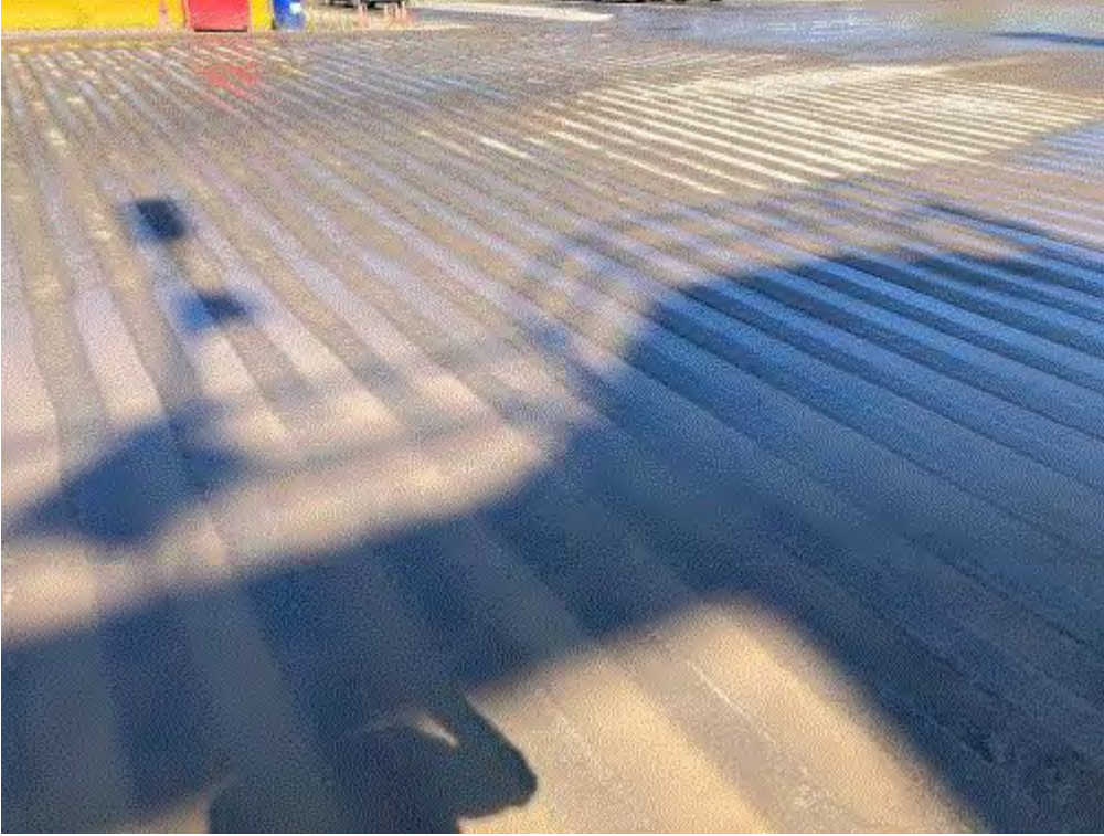
Image 1(001) : Rumble strips which have been watered to enhance effectiveness.
