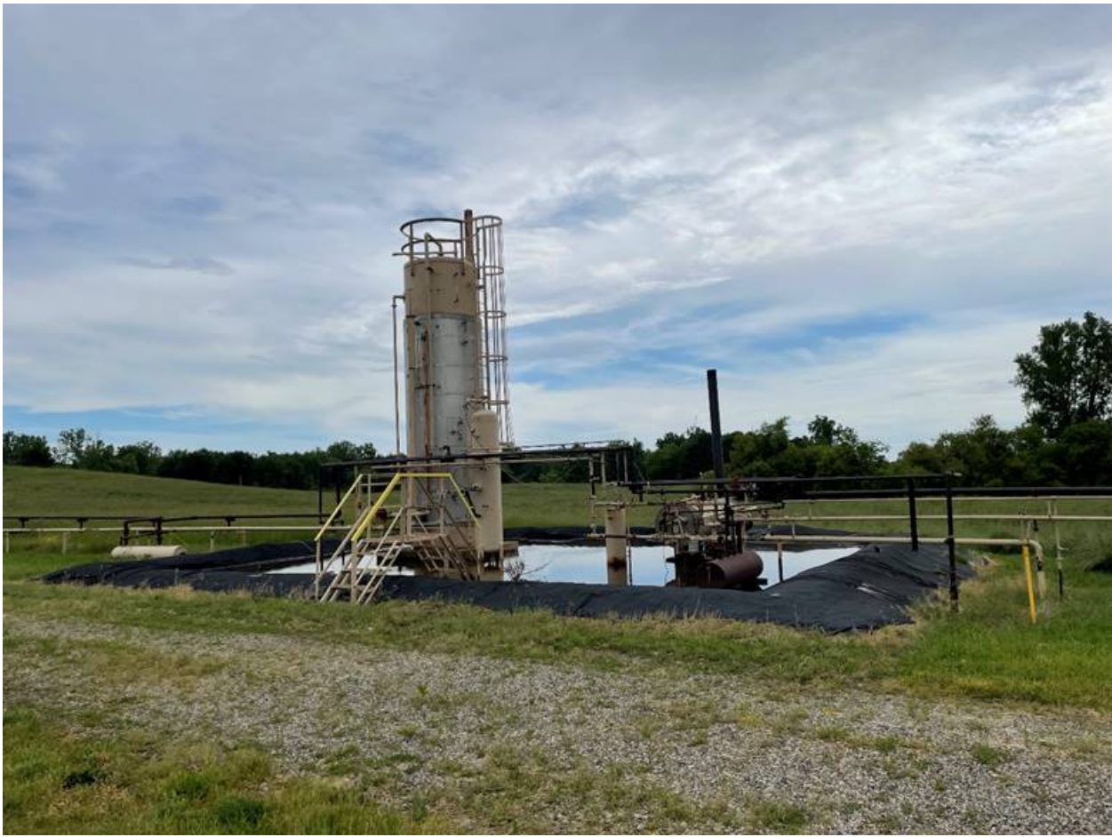
Image 3: Wessel 1-6 heater treater and line heater.
