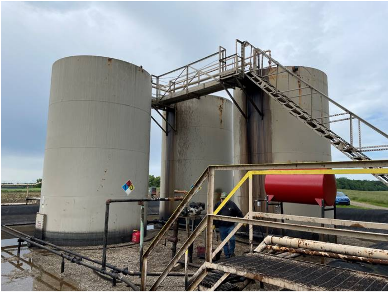
Image 6: Wessel 2-6A storage tanks. Note stained sides of tank.
