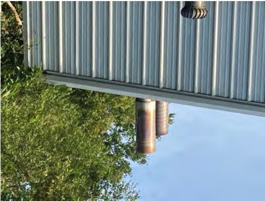
Image 2(Stacks) : Stacks for both burnoff ovens
