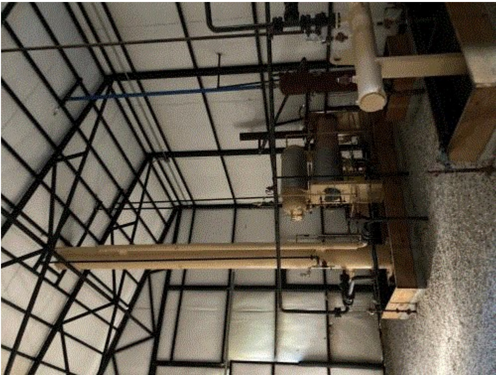
Image 3(Dehy Unit) : Tower has a PSI of 1100; Heater was not working. Notice short stack on Dehy.
