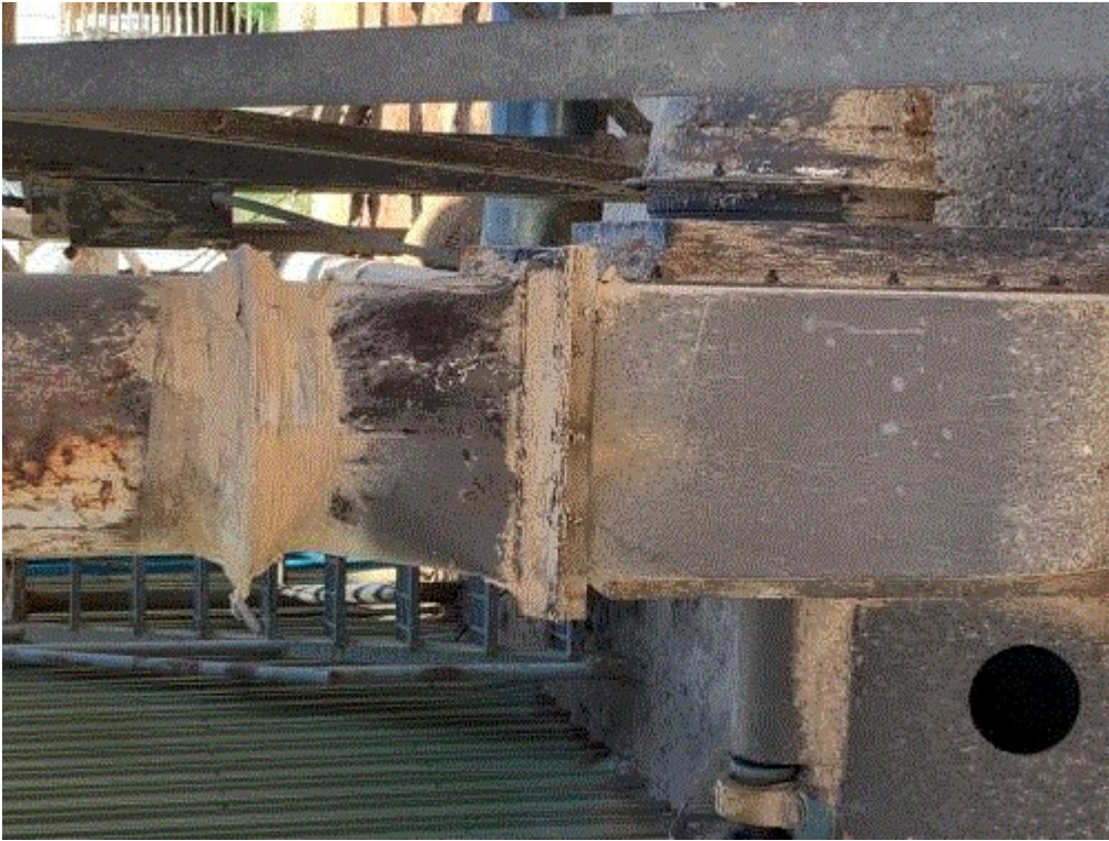
Image 8(South Baghouse) : Hole in ducting and ducting flange connection wrapped in plastic.
