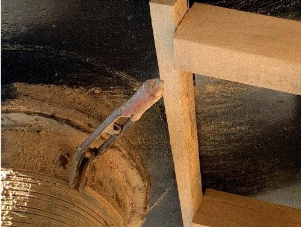
Image 10(South Baghouse) : Broken collection bin to ducting clamp.
