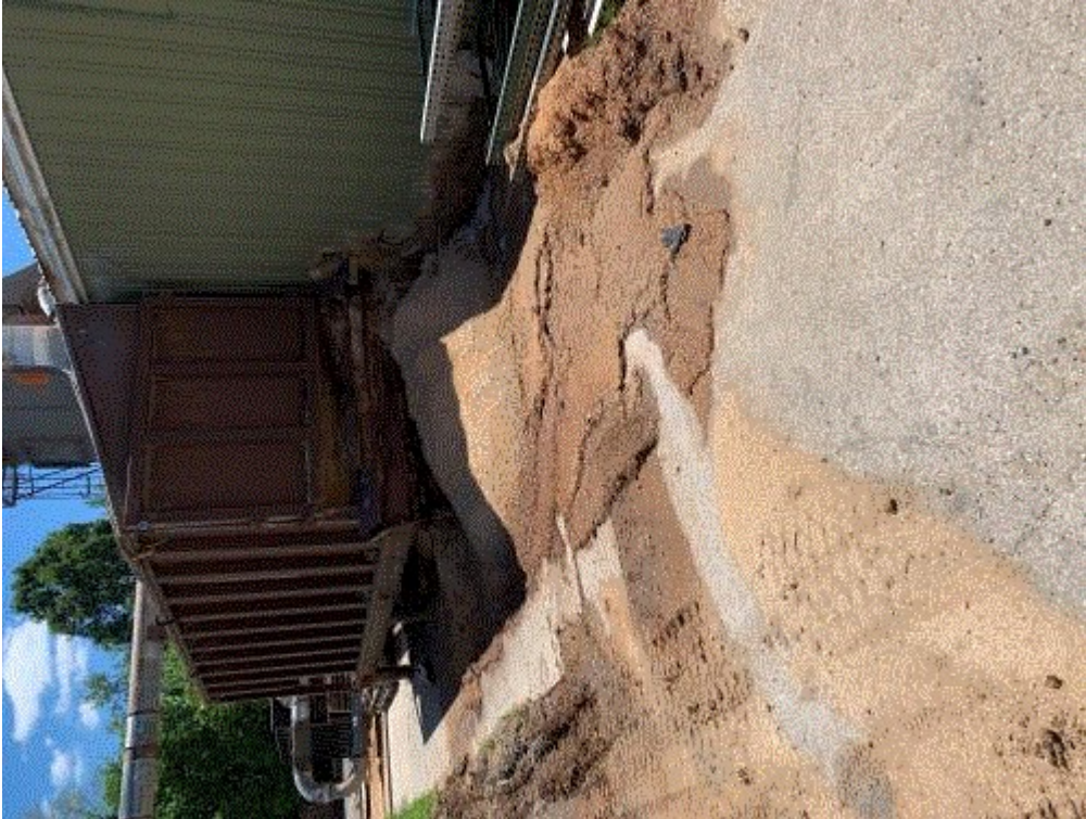
Image 1(South Baghouse) : Wood waste furnace collection bin and auguring system.
