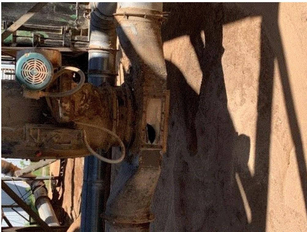
Image 7(South Baghouse) : Hole in blower access cover.
