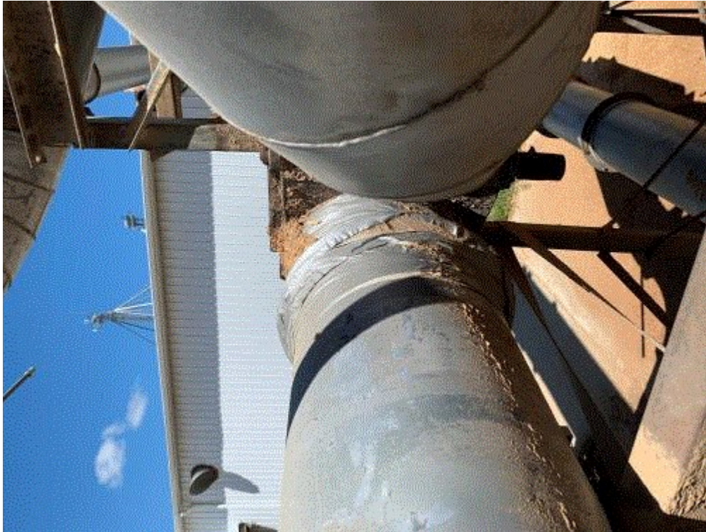
Image 6(South Baghouse) : Ducting joint flange wrapped in duct tape
