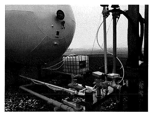
**Image 3(003):** Yellow vapor return lines and orange liquid lines with check and flow valves.
