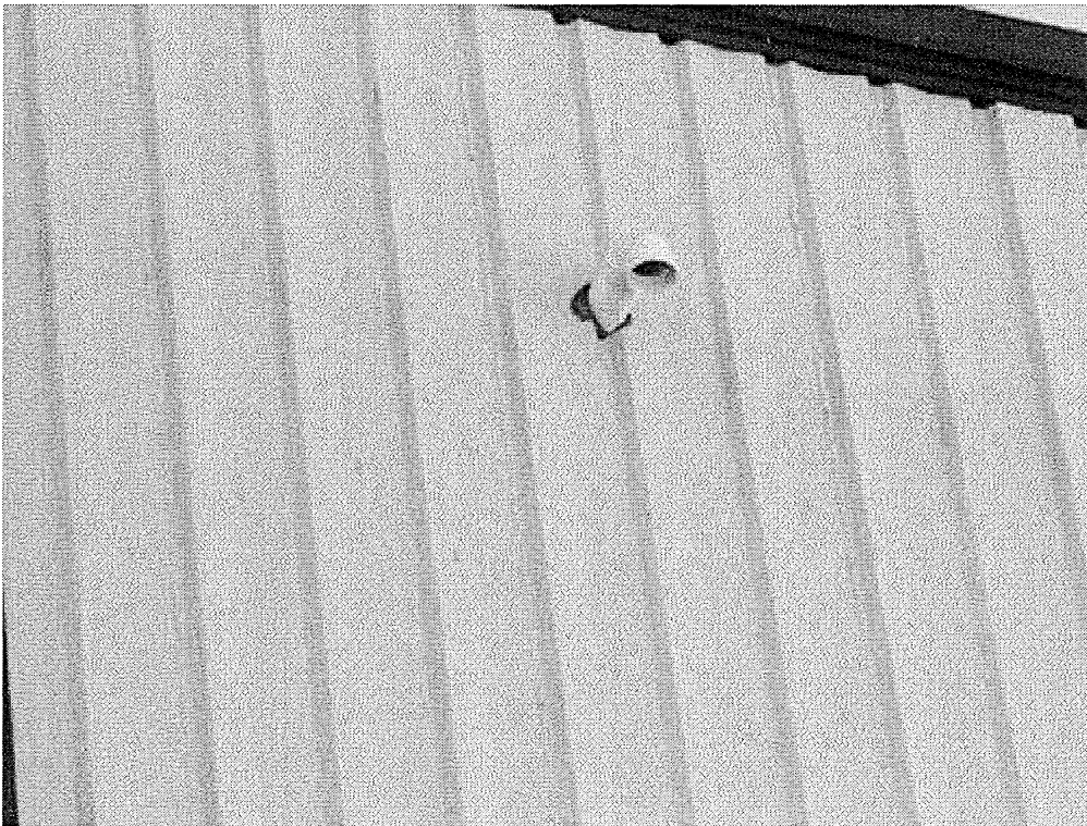
Image 2(Small exhaust) : Small exhaust going out side of building on the West side. It contains water vapor and methanol from the front dryer skid pump that is part of the enzymatic process flow
