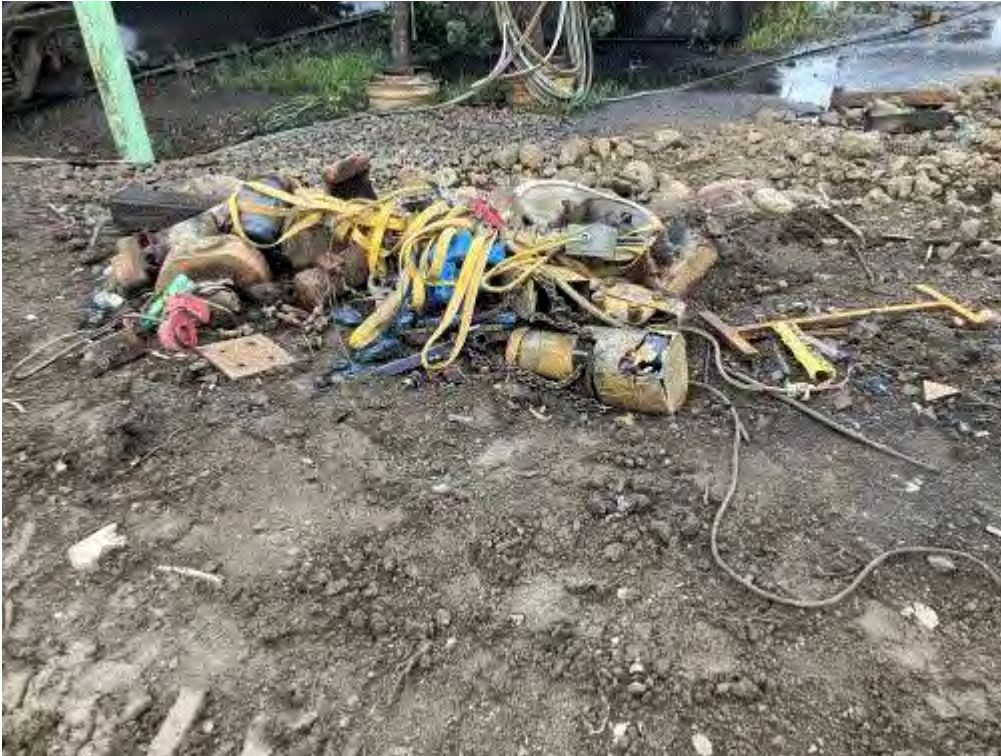
Image 9(009) : More materials removed from steel scrap prior to torch cutting, including electrical system components.
