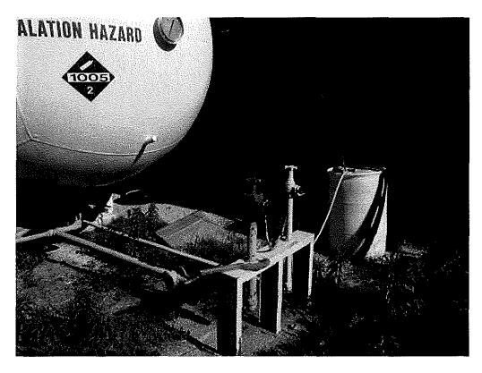
Image 1(Bulkhead): Permanent storage tank bulkhead, water trap, and safety valve
