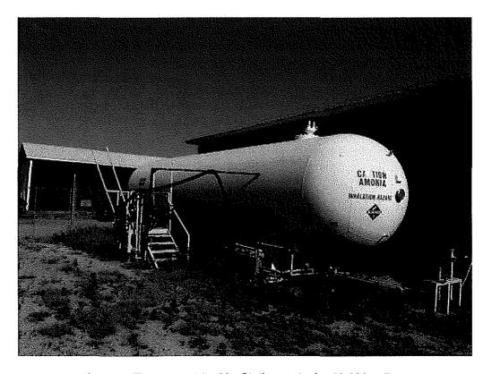
Image 5(Permanent tank): Stationary tank - 18,000 gallon
