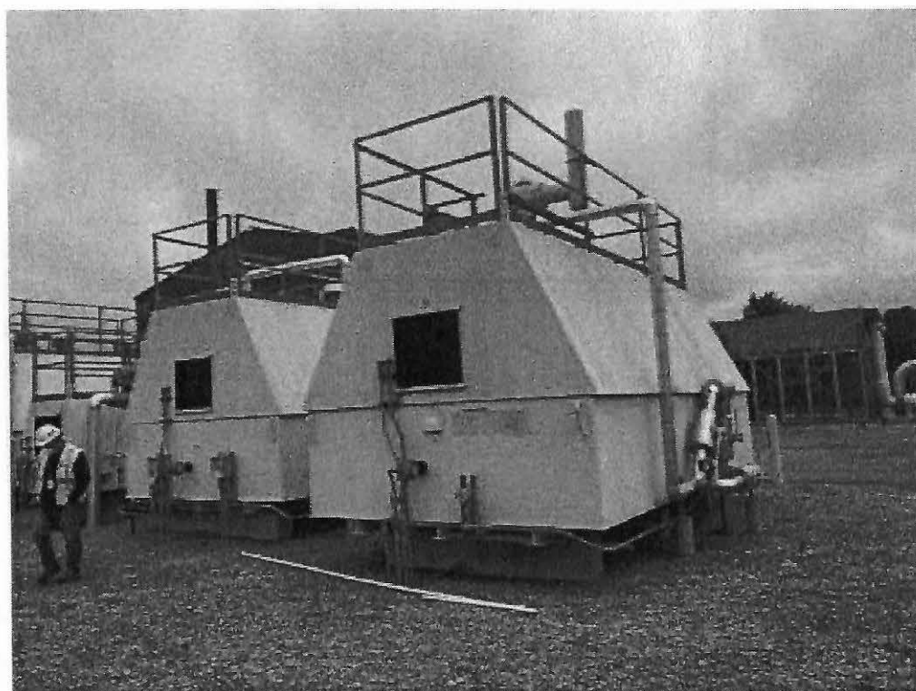
Image 2(5000 gallon tank) : 5000 gallon tank(on right) that had greater than 600,000 ppm methane leak coming out the top.
