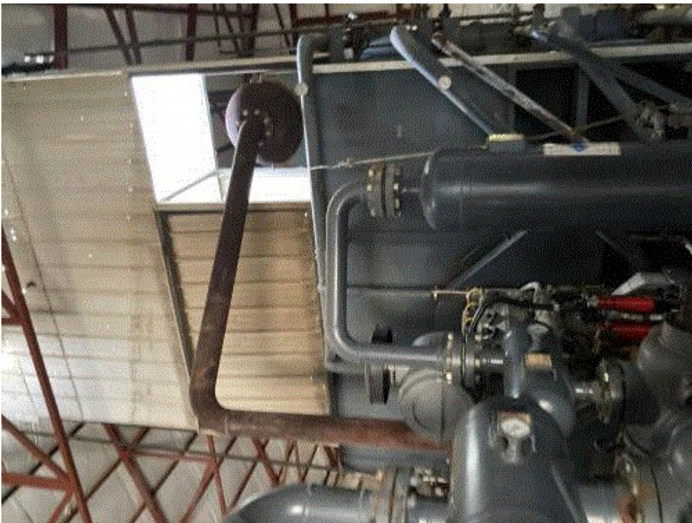
Image 5(Stack) : Stack going to Muffler with no Catalytic Control
