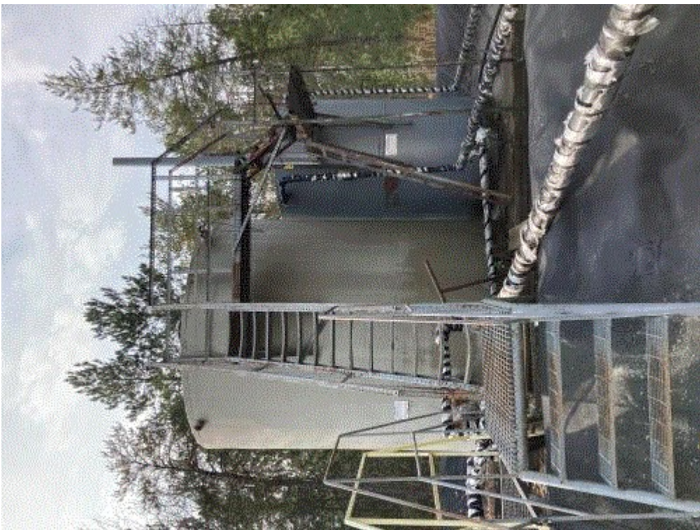
Image 3(AST Tanks) : 1 - 400 BBL Brine Tank & 1-200 BBL +/- Slop Tank.
