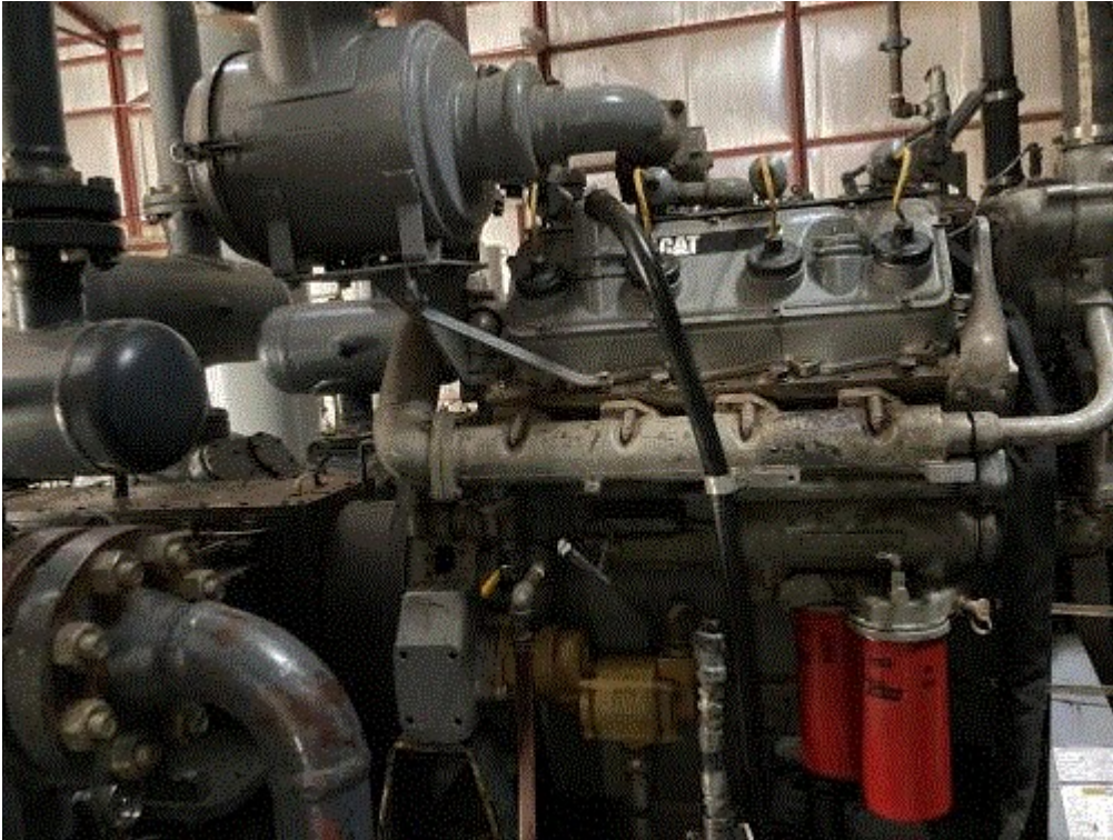
Image 6(Engine) : 8 Cylinder Engine
