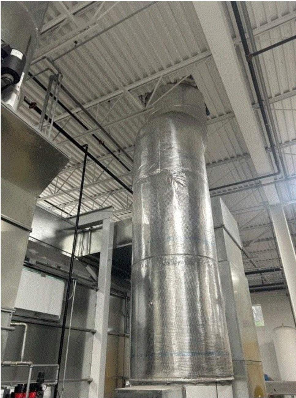
Image 5(Coating booth vent) : Coating booth internal venting system
