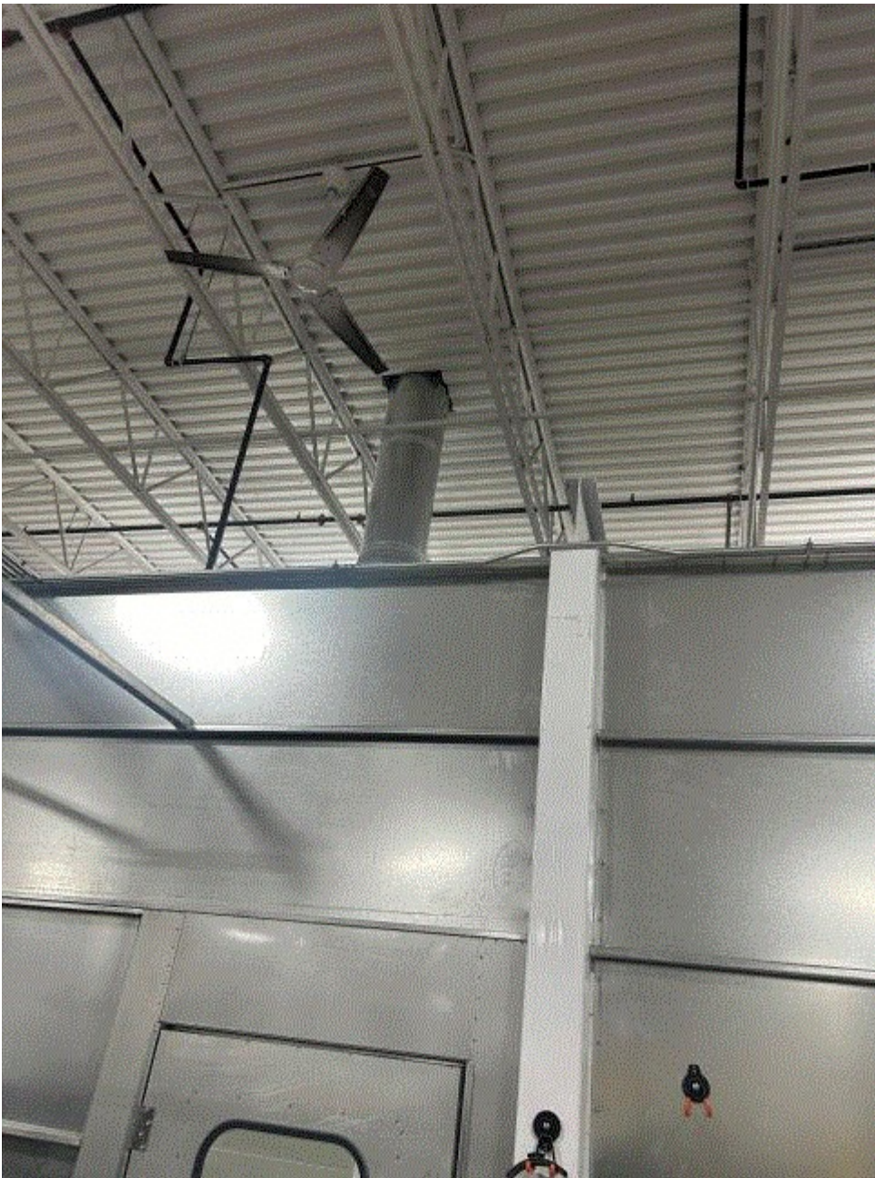
Image 6(Dry booth vent) : Internal dry booth ventilation system
