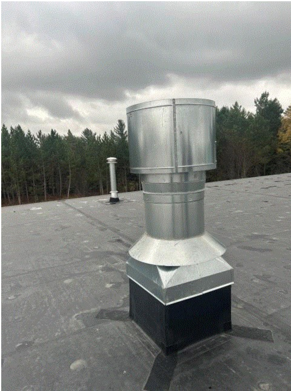
Image 4(Sanding booth roof) : Sanding booth roof vent
