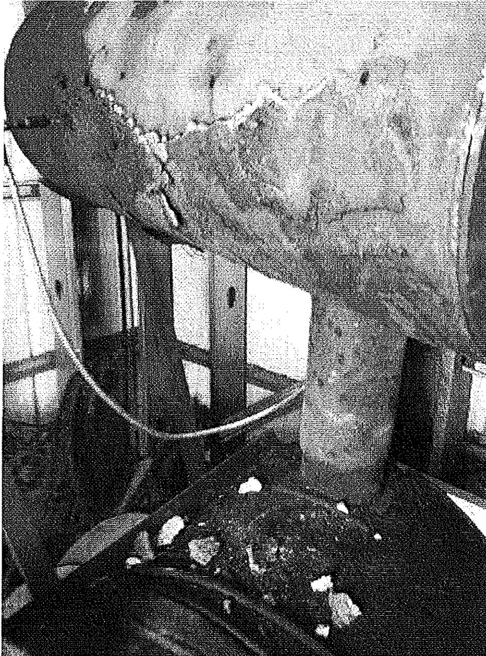
Image 4(ccvc4) : jacket disintegration on afterburner
