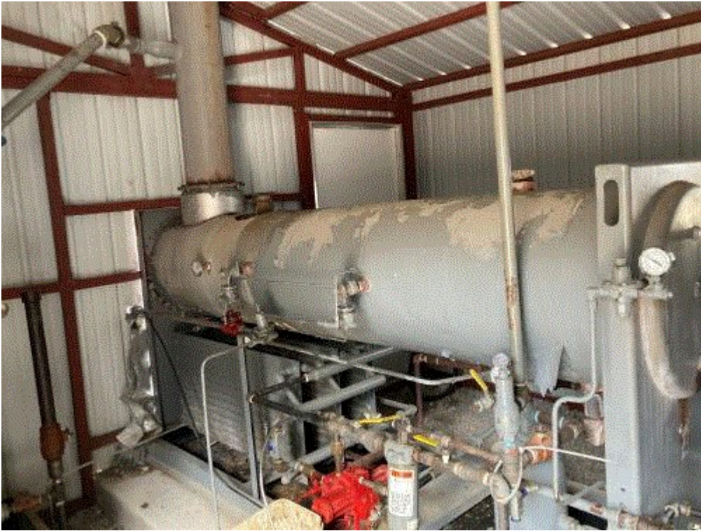
Image 8(Dehy Reboiler) : Reboiler was operating at 250 Deg F.
