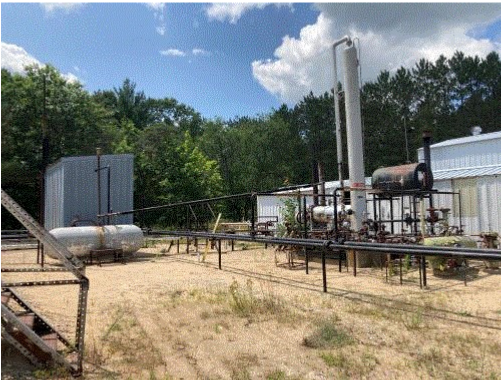
Image 2(Dehy & Separator) : There were low odors coming from the Dehy unit and the vent from the 500 gallon
