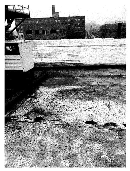
Image 2(EUBASECOAT #2.2): Improper control of paint particulate.
