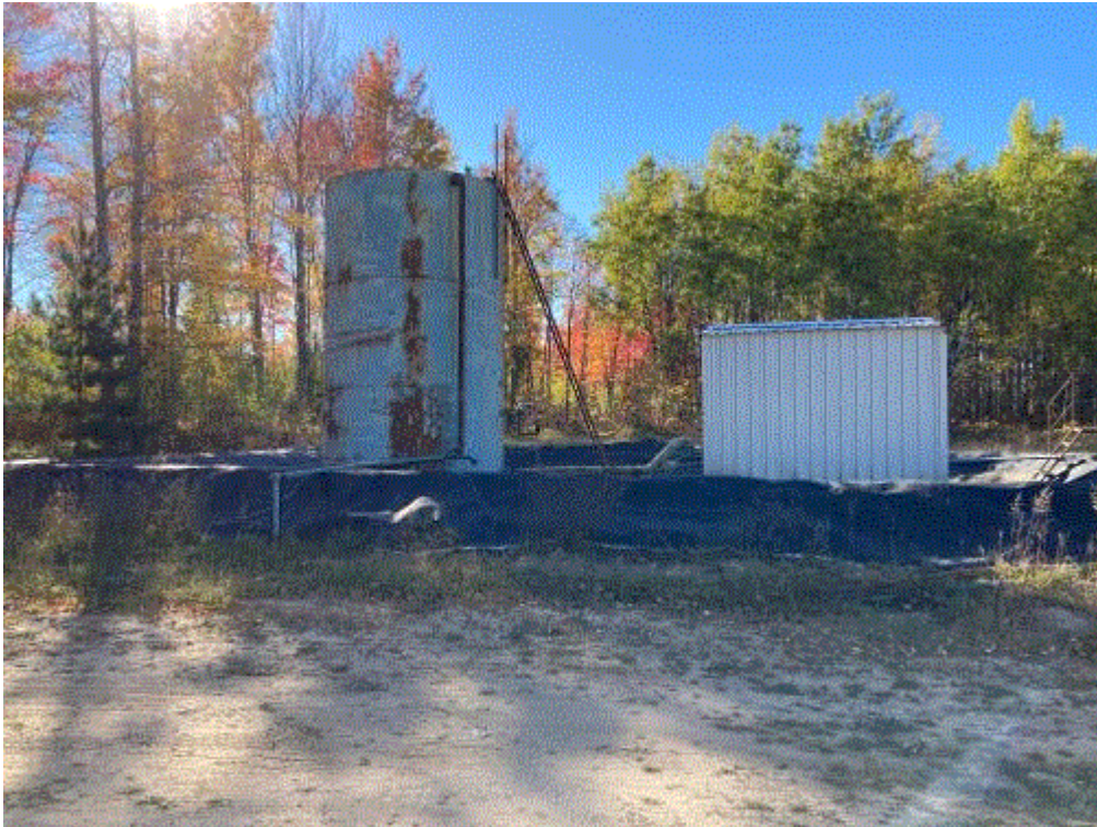
Image 3(400 BBL Tank) : AST Tank and Shed
