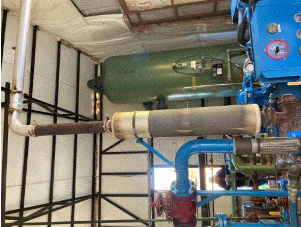
Image 5(Engine Stack) : Engine Stack with Muffler
