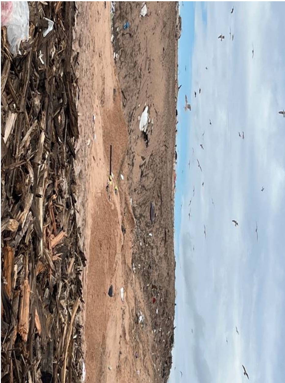
EUASBESTOS asbestos waste hole. Breaks in cover are visible.
