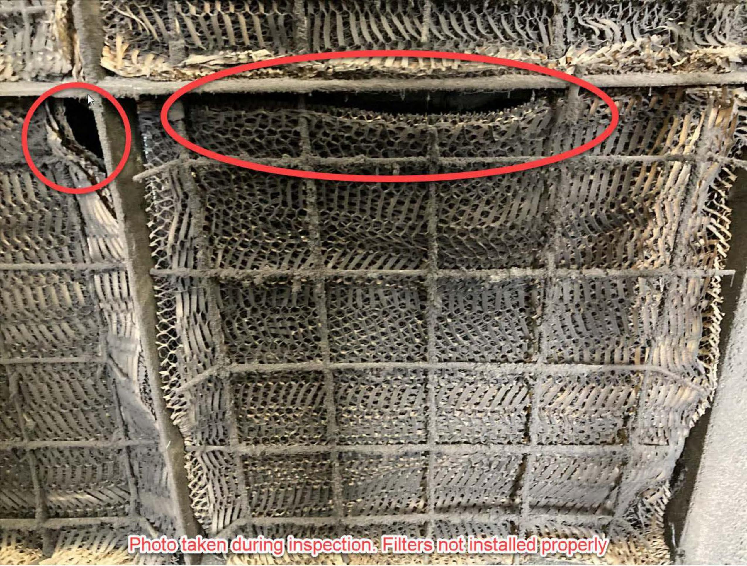
Photo taken during inspection. Filters not installed properly
