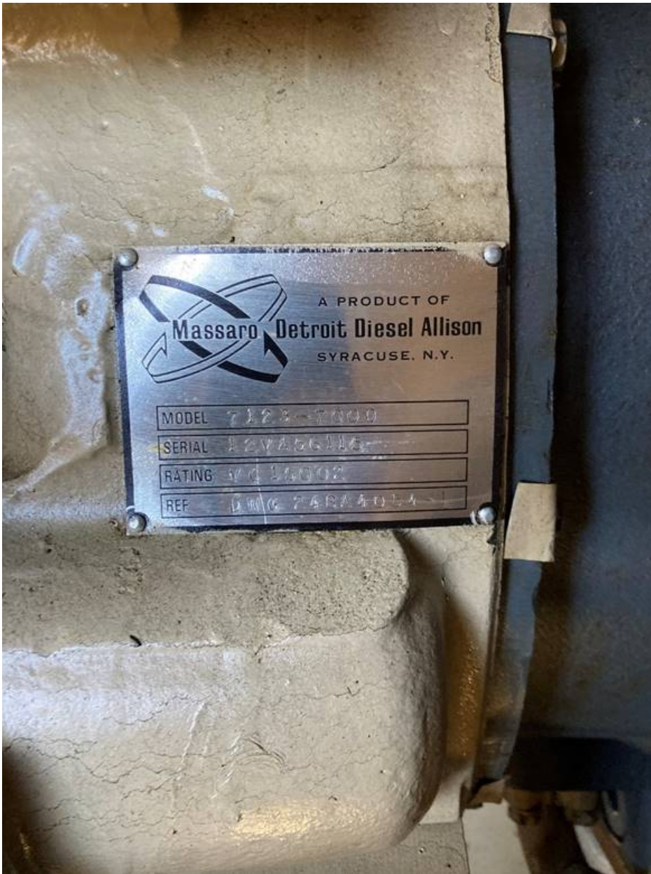
Image 3: Black start engine name plate
